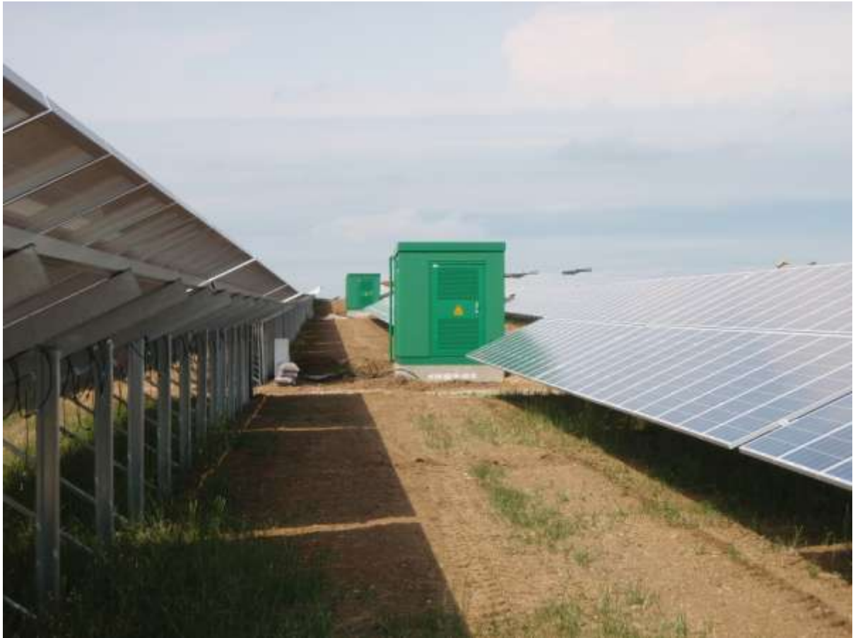
Plate 7. Inverter bases completed (looking west)
