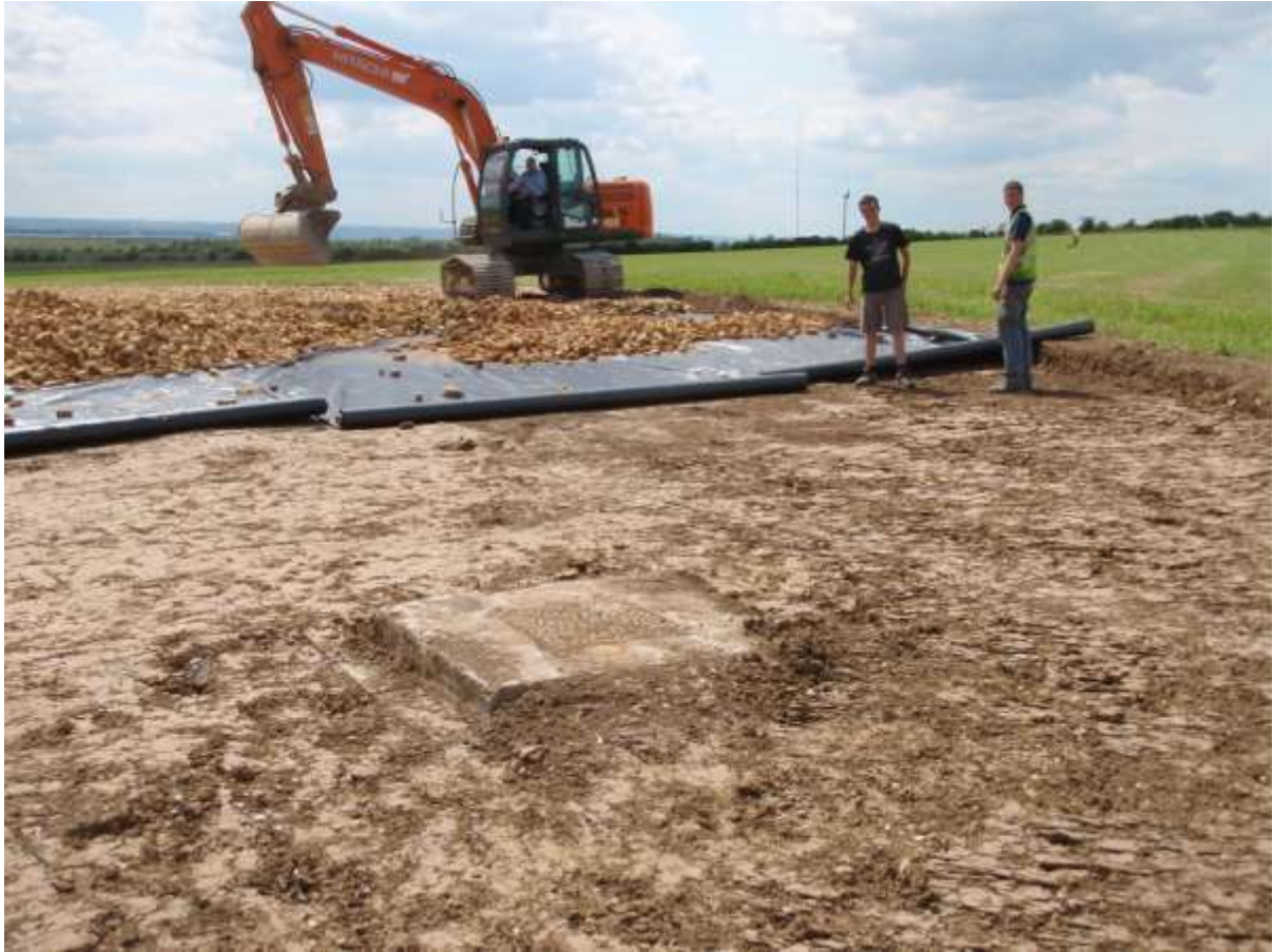
Plate 2. Access road construction with ditching bucket (looking south-east)
