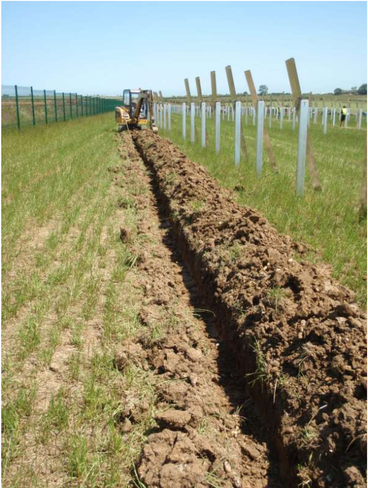
Plate 5. Cable runs between solar panels (looking east)
