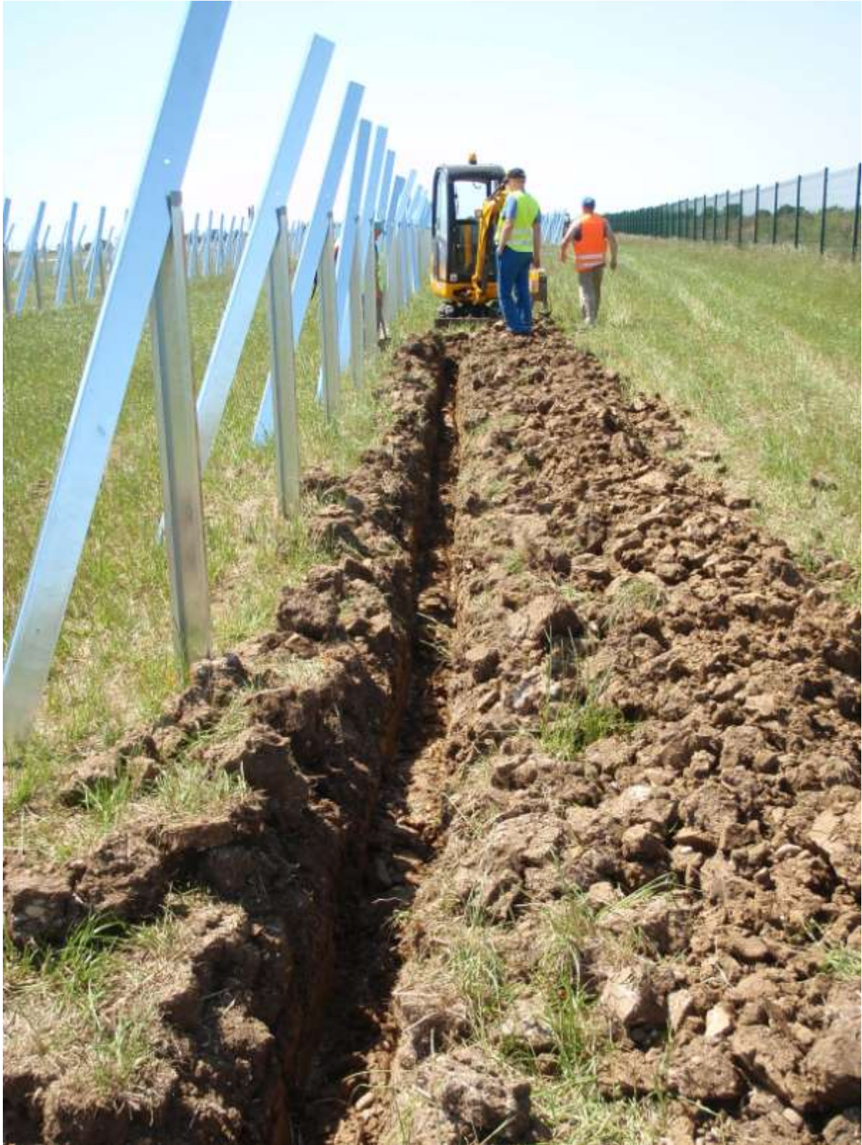
Plate 4. Cable runs between solar panels – security fencing seen to the right (facing west)
