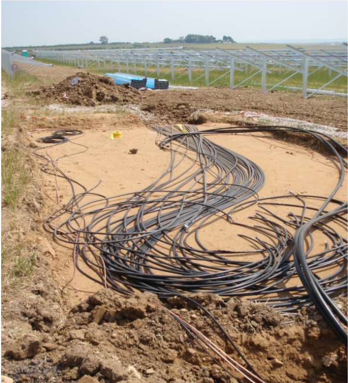
Plate 6. Cable runs to inverter bases (looking east)
