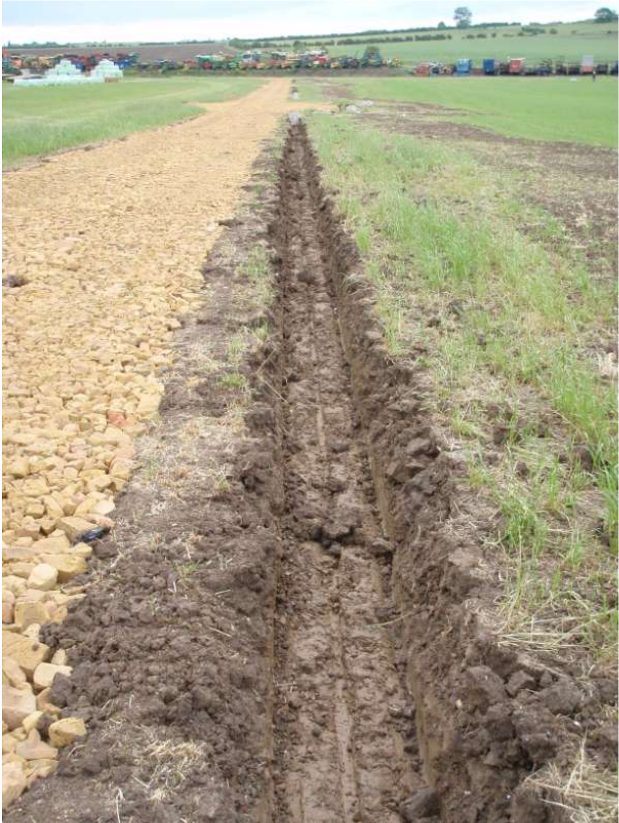
Plate 3. HV Cable runs to inverter housings (looking east)
